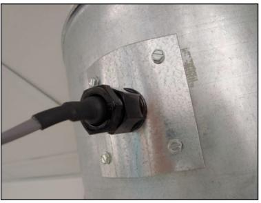
The intended application is for use with bio-safety cabinets. The probe is installed in the exhaust duct above the cabinet's transition collar with a provided mounting plate, a 3-by-3-inch galvanized steel square (see picture at left). The sensor holes should be positioned in the direction of the airflow. The sensor works best when installed in the center of the duct. If it sits just on the edge of a duct it may sense turbulence. If it cannot be repositioned, a longer tube may be a solution.
